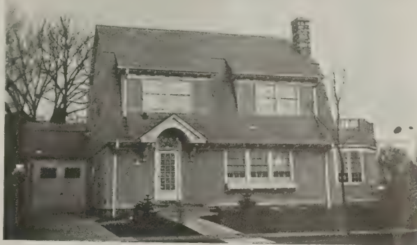
FIG. 2. GARAGE BUILT AS WING OF HOUSE, BUT SET BACK SO AS TO PERMIT THE PROVISION OF WINDOWS IN SIDE WALL OF HOUSE PROPER
